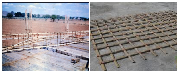
Fig. 7: Construction Site used Bamboo.
